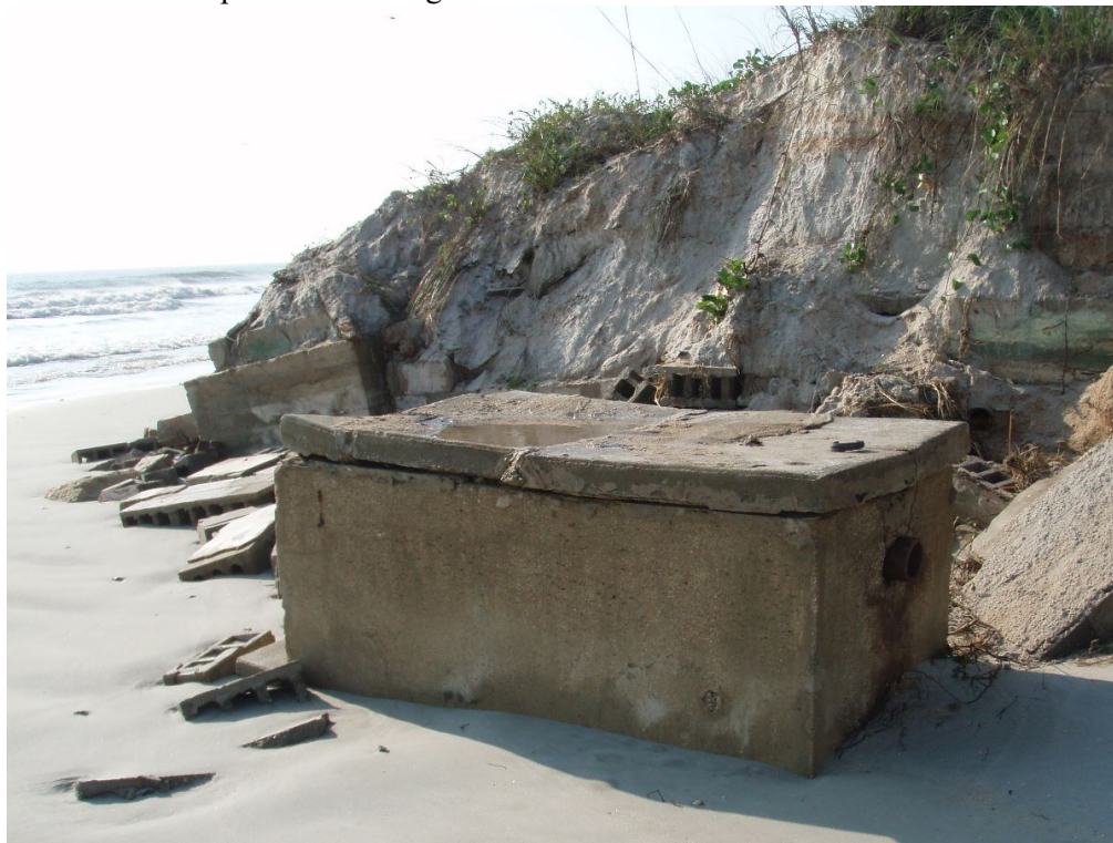
Figure 5. Septic tank exposed by coastal erosion. Credit Miami-Dade County.
