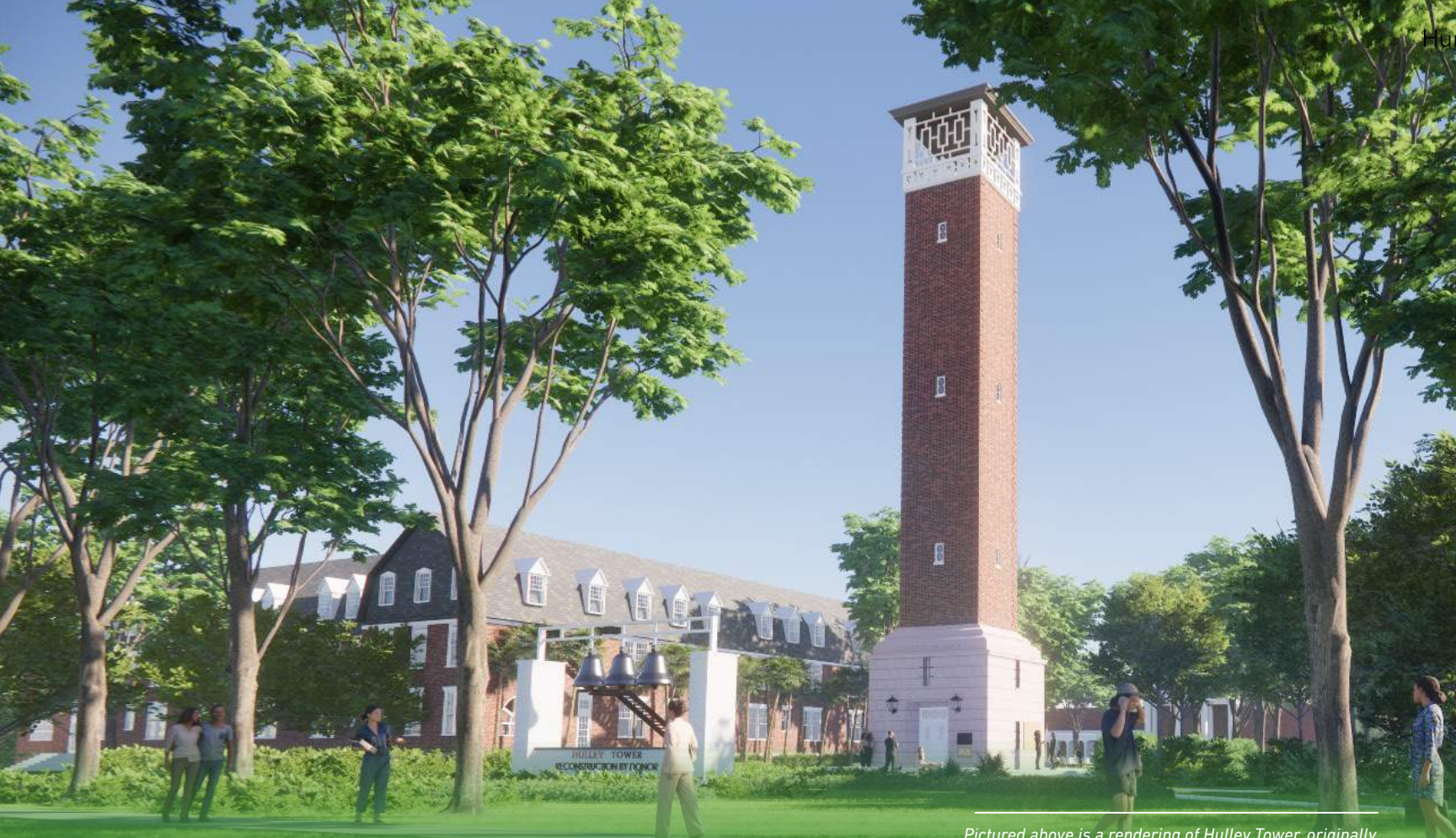
Pictured above is a rendering of Hulley Tower, originally built in 1934, undergoing a historic reconstruction to restore its 116 ft. height and new 52 bell carillon. This landmark at the Stetson DeLand campus will once again inspire our community to remember, reflect, connect and engage in the Soul of Stetson.
