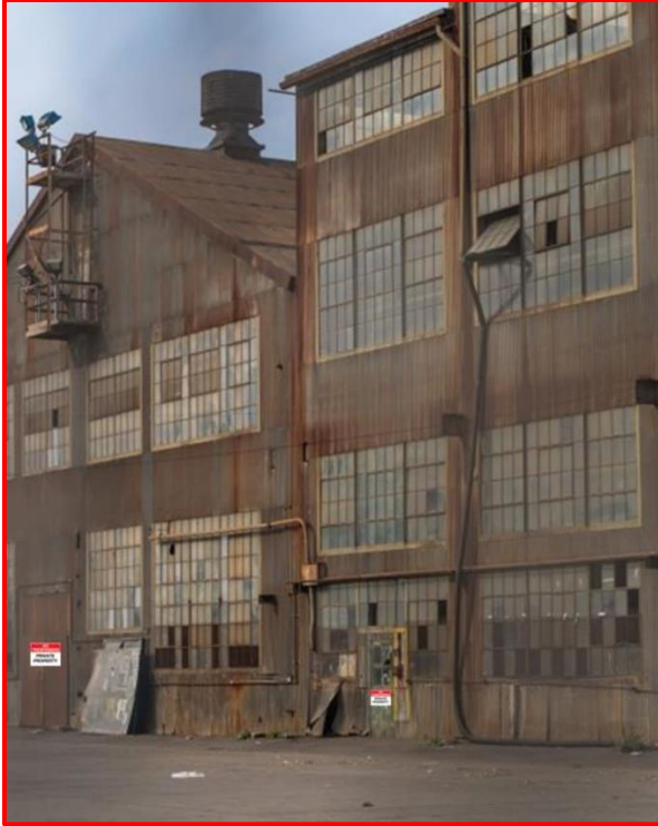
Warehouse Exterior (Ex. 4)
