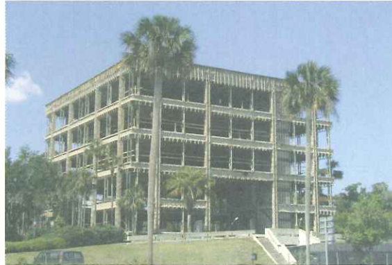
Under Reconstruction – 2001 Photo by Lynn Thompson
