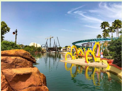
A view of construction on VelociCoaster, 2020
